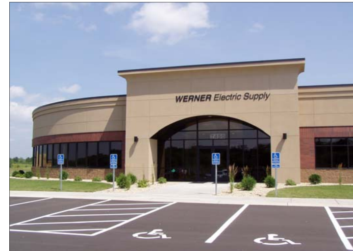
Completed Werner Electric Supply Facility
