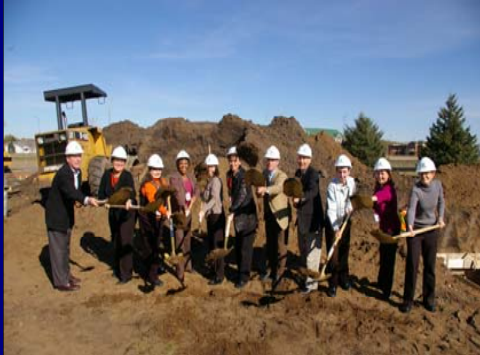
Allina Expansion Ground Breaking
